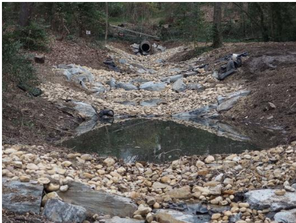
Fig 9-5 Stepped Pool Conveyance System: NPV
