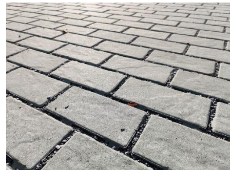
Fig 9-4 Interlocking permeable pavers, Source: NPV
