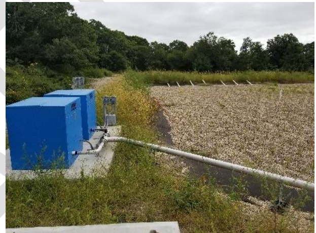
Fig 9-6 Constructed Wetland ,Source: NPV
