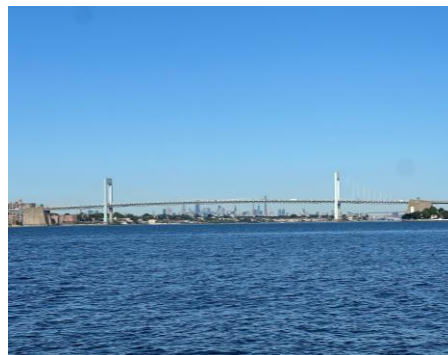
View of Manhattan behind the Throgs Neck Bridge during Survey #2
