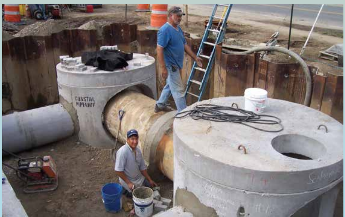
A newly installed filtration system prevents sedimentation.
