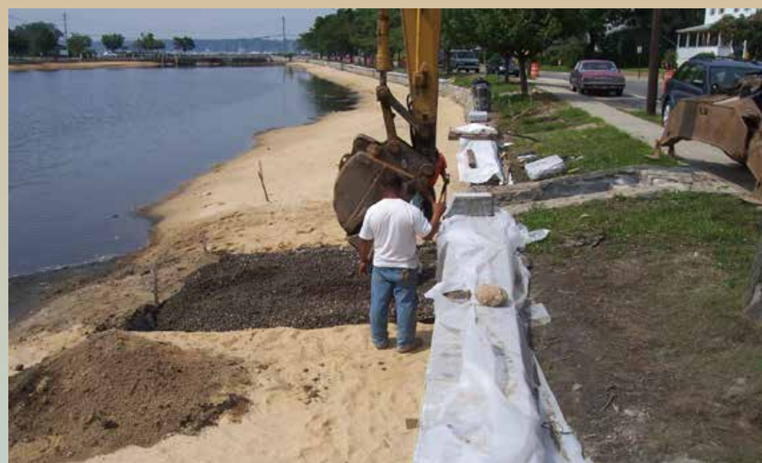
Extensive reconstruction of the pond wall
