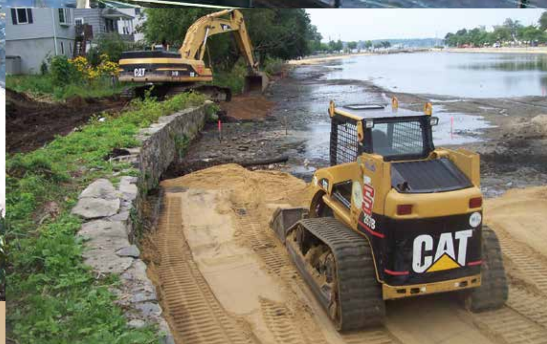
Heavy equipment reshapes the pond's perimeter.
