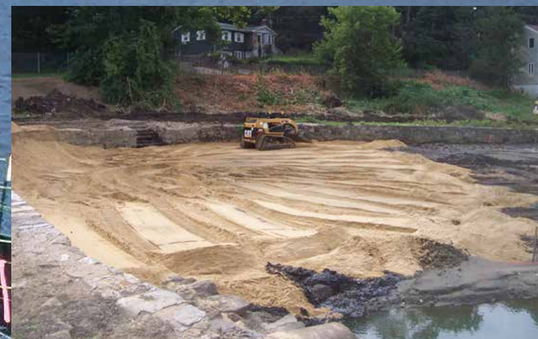
Pond floor is regraded, dredged, and cleaned.
