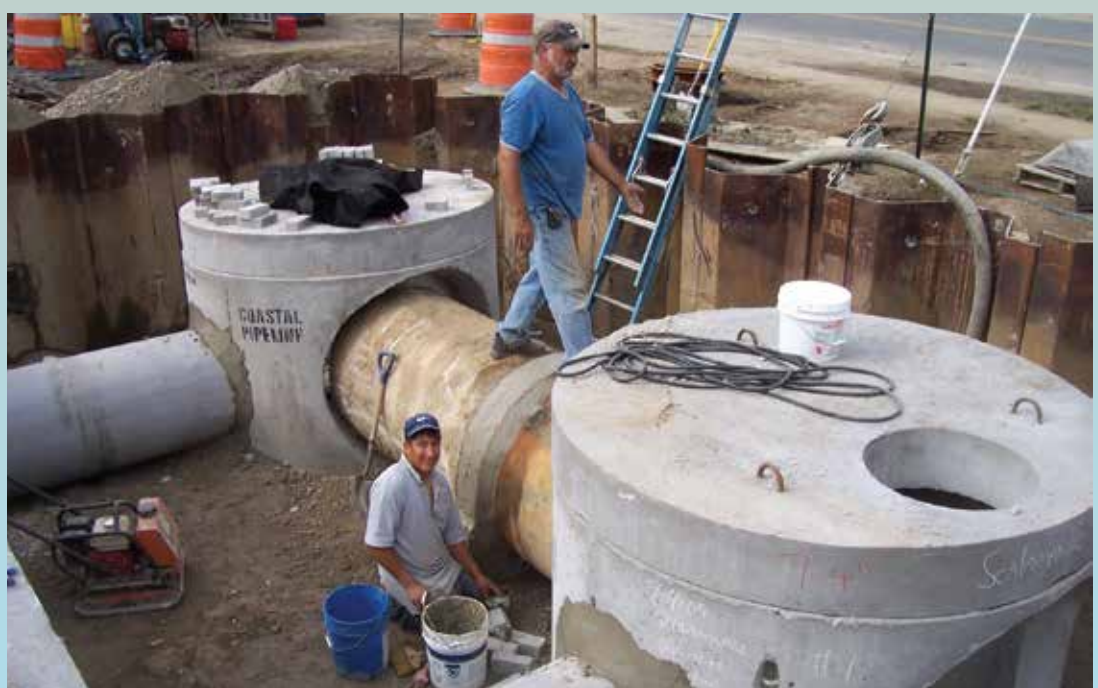
A newly installed filtration system prevents sedimentation.
